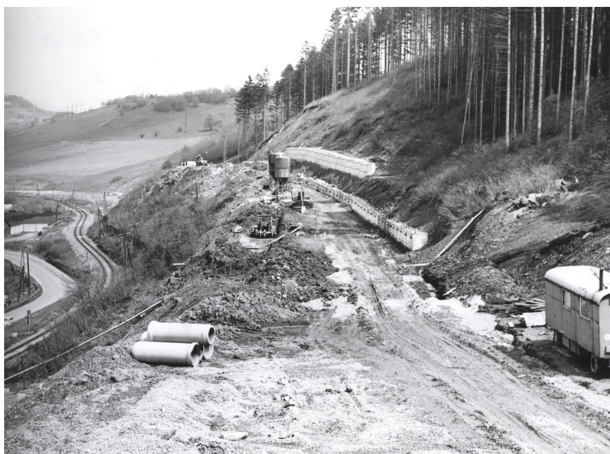
Fig. 12. Stabilization works on the landslide caused by undercutting on the highway near Dolný Kubín town (North Slovakia – Photo J. Malgot)
