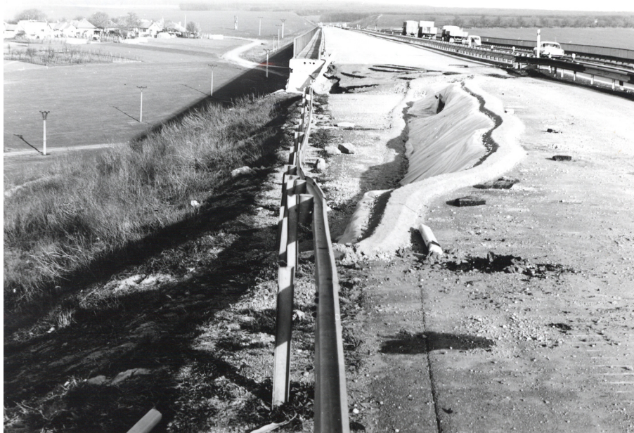
Fig. 3. Failure of the body of a highway embankment near Nitra town (Photo J. Malgot)
