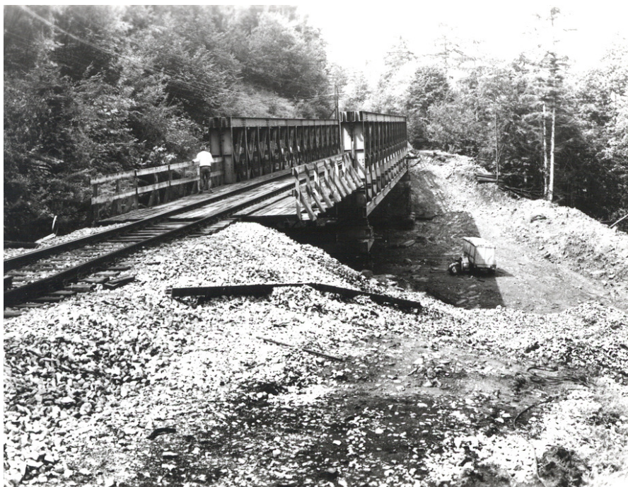
Fig. 5. Activation of landslide after construction of railway embankment near Kremnica town (Photo J. Malgot)
