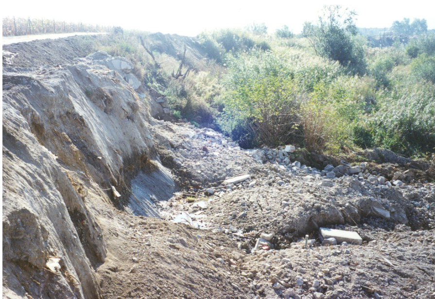
Fig. 6. View of slide on the body of dump in Bratislava (Photo J. Malgot)
