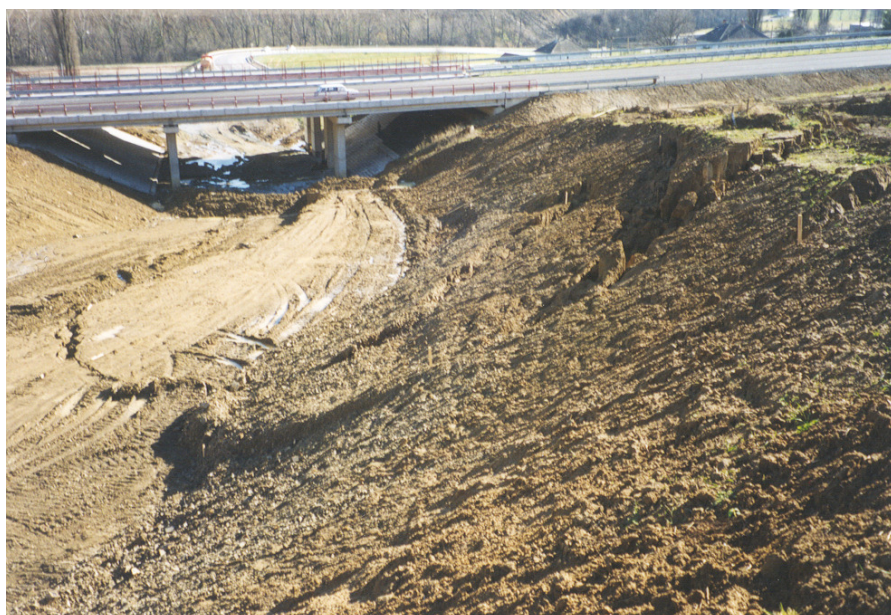
Fig. 10. View of a landslide caused by undercutting of a dormant landslide near Prešov town (Highway D1 – Photo J. Malgot)
