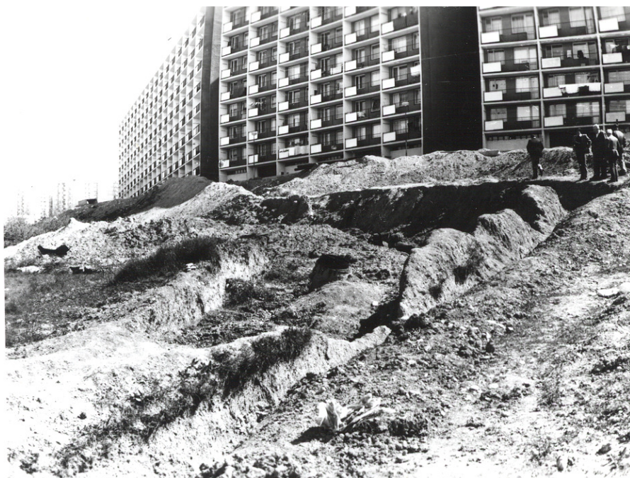
Fig. 9. View of a landslide evoked by undercutting of a slope in a new part of Košice town (Photo A. Nemčok)
