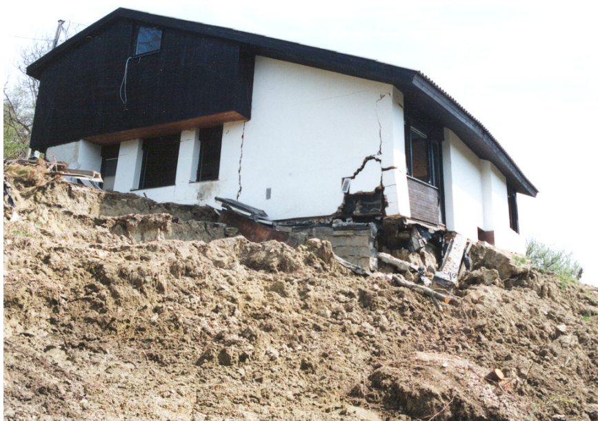
Fig. 16. Destroyed house by landslide near Košice town (Photo F. Baliak)
